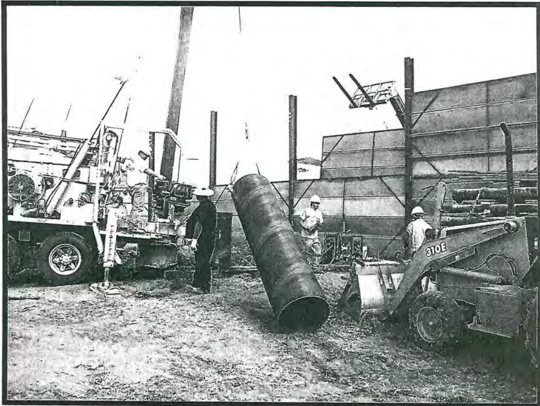
Installing 36-inch conductor pipe
