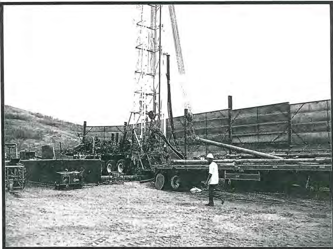
Drilling 24-inch pilot hole
